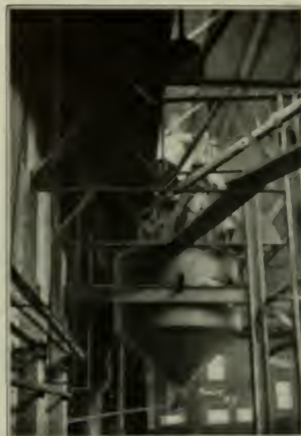
FIG. 3. STEEL STORAGE TANK AND SETTLING CHAMBER ABOVE
